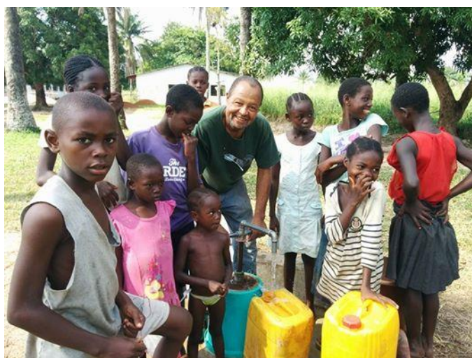
Following the success of Leon's first month of work on the latrines and rainwater catchment tanks, the project was amended to include several wells in lieu of the sand filters in the classrooms. Here the first well is issuing fresh clean water.
